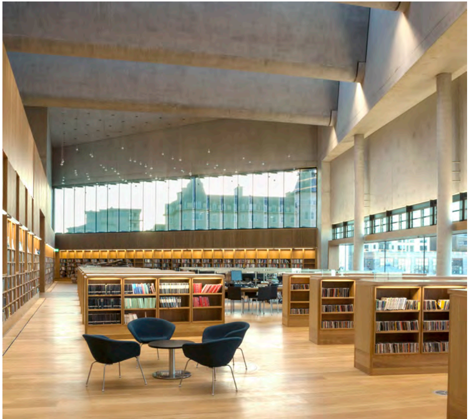
ABOVE The concrete mix used at the DLR Lexicon library in Dún Laoghaire, County Dublin, includes 50% GGBS
