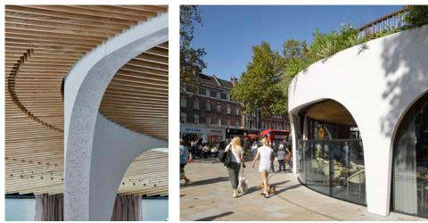
We chose a white concrete, with an off-white fine aggregate of quartz and a coarse aggregate of dolomite. The front and back surfaces have been acid-etched to give a slight lustre to the quartz – with curved concrete, you really want to do as little finishing as possible. But within the arches, we heavily ground and polished the reveals to show the pale-grey and blue dolomite stones. Conceptually, it reinforces the idea of a continuous ribbon being cut to form these openings.
