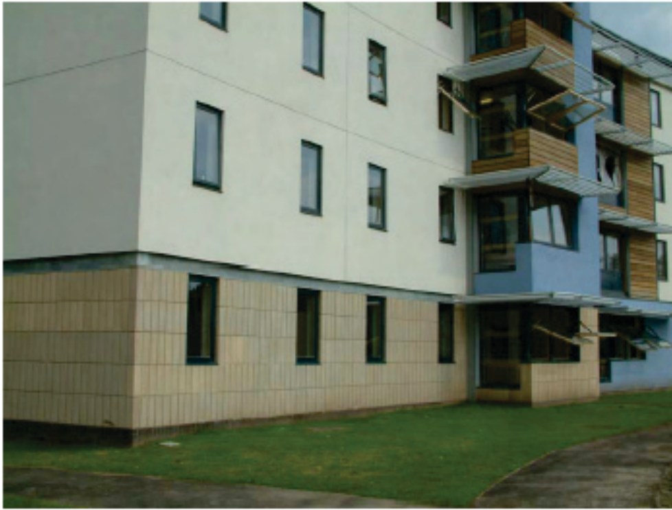
Colman House Flats 28 & 30 Test Elevation Rooms A - C
