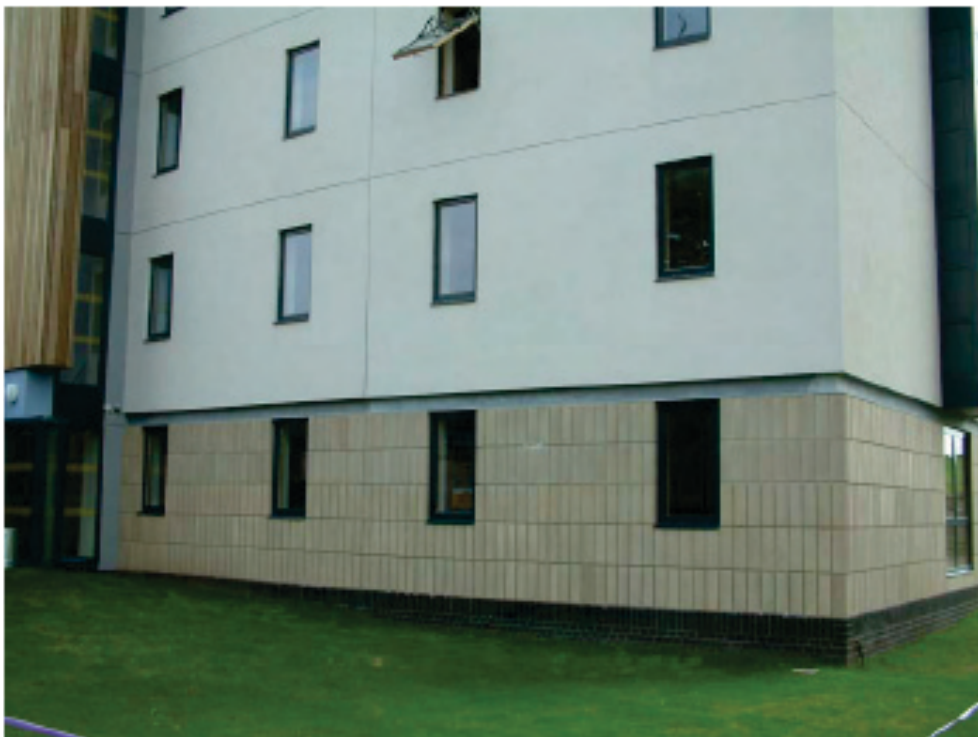
Colman House Flats 28 & 30 Test Elevation Rooms F - H
