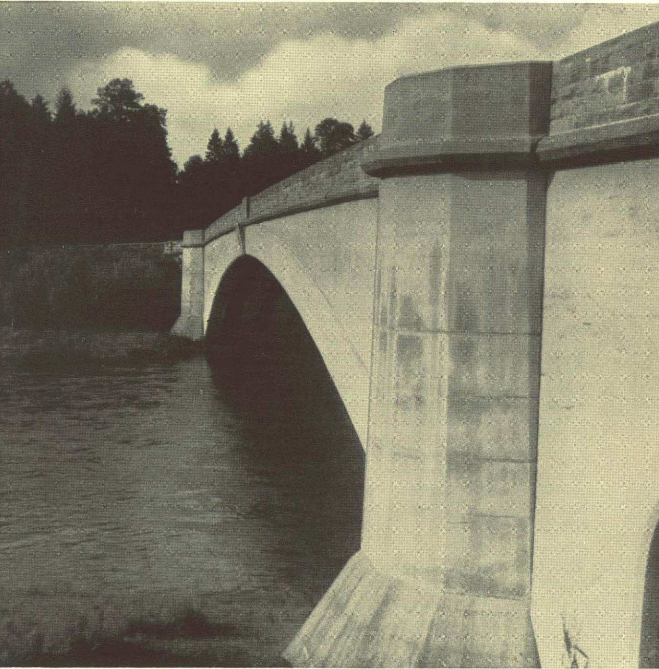
The Spey Bridge at Granttown which links Moray and Inverness. Engineers : Blyth & Blyth, MM.I.C.E.
