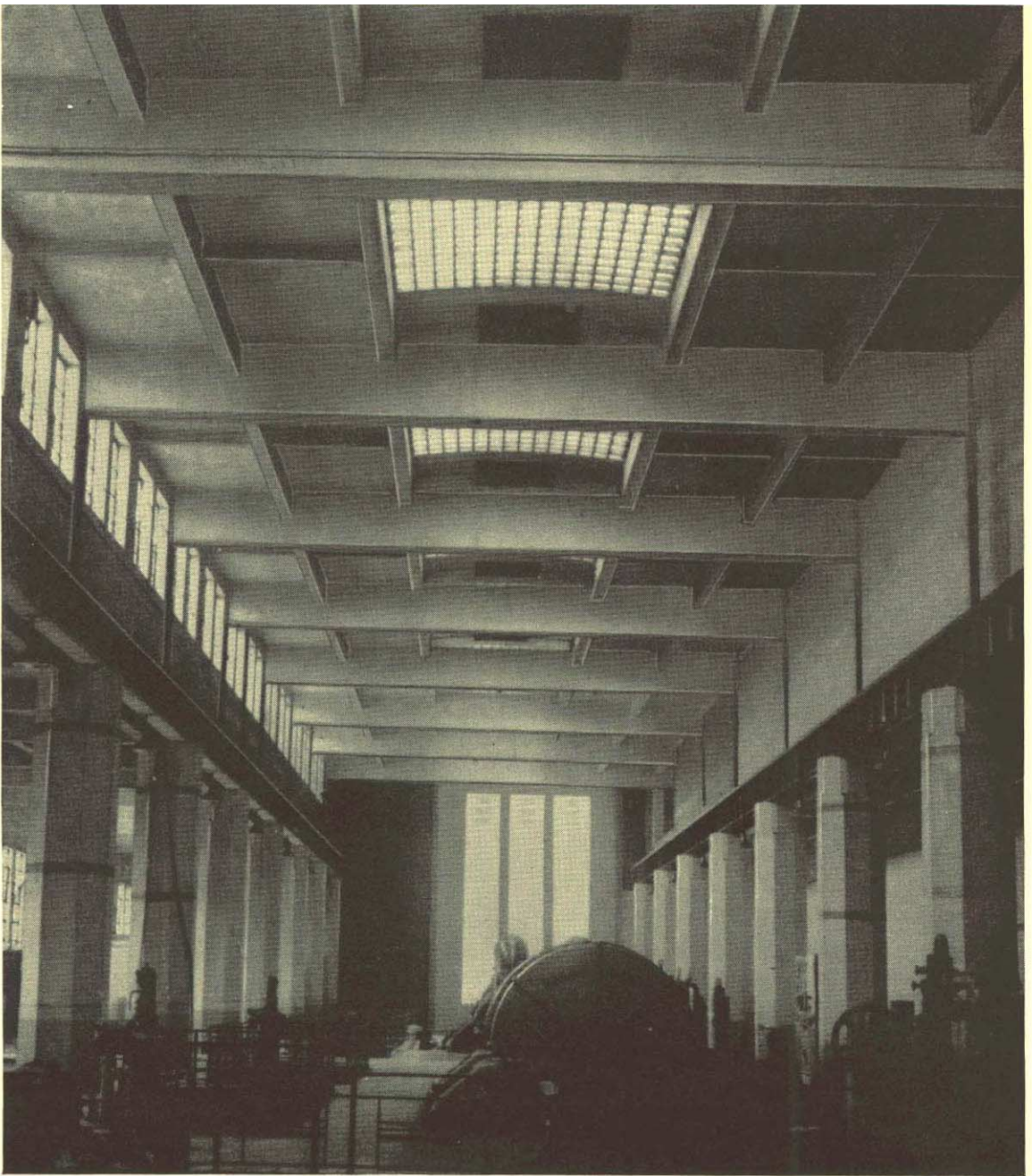
Interior of turbine house showing Lenscrete roof lights.
