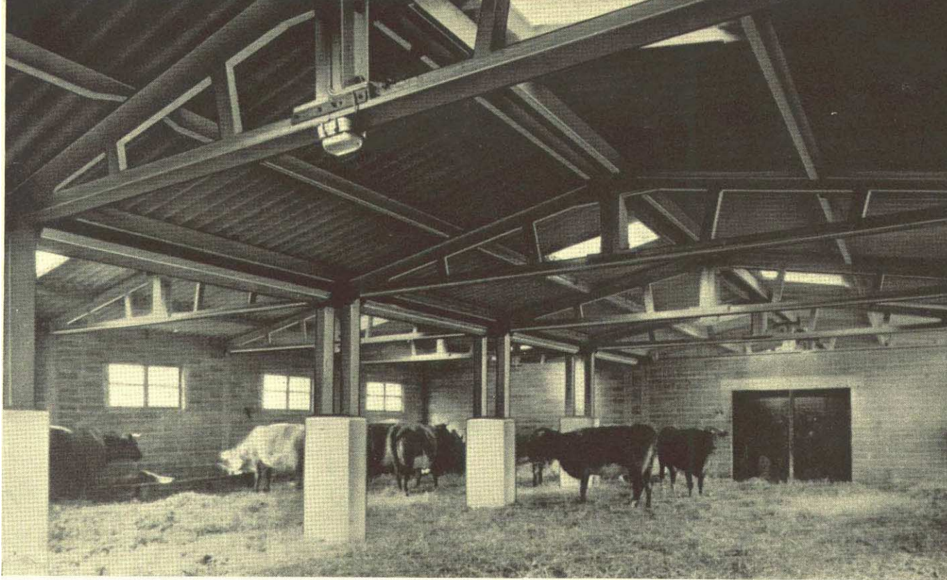
A covered stock-yard 80 ft. long and 40 ft. wide. The roof is constructed with 20 foot span precast reinforced concrete roof trusses, supported on precast reinforced concrete columns. The centre columns have a protective casing, also of concrete, with rounded corners as a safeguard for the cattle rubbing themselves. The roof is covered with corrugated asbestos cement sheets. The concrete floor slab is 6 in. thick. (The Home Farm, Thornborough, Bucks.).
