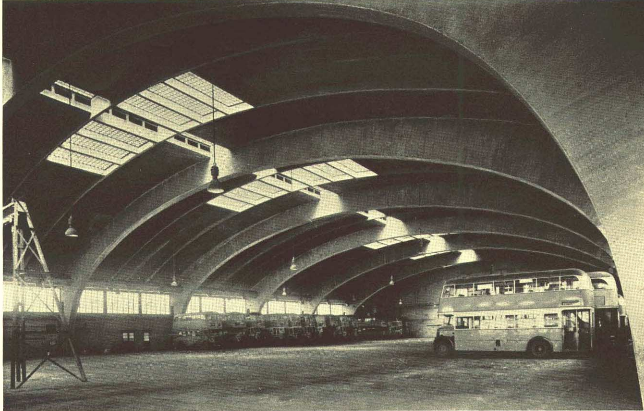
ABOVE: The unobstructed garage floor, providing accommodation for 100 buses.
