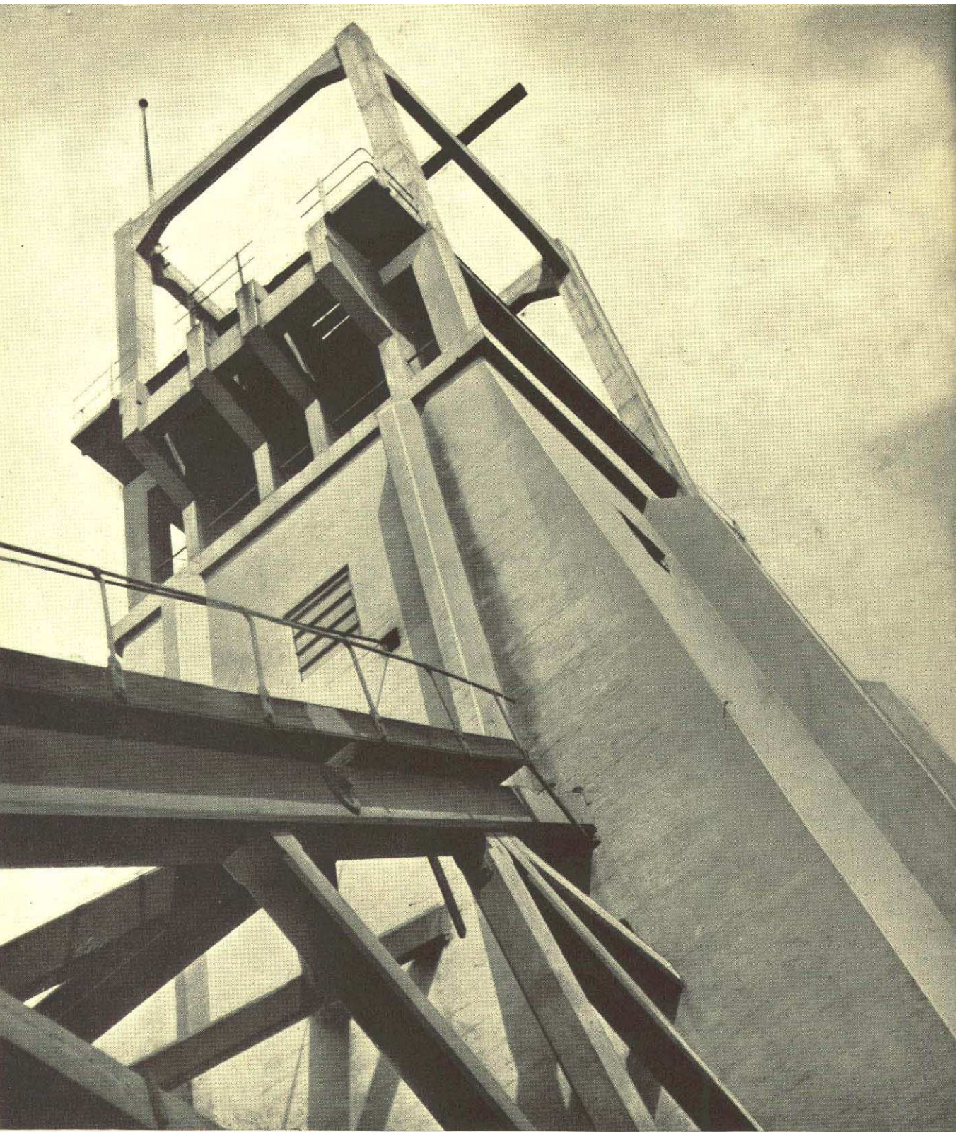
New headgear and airlock, showing the struts supporting the old steel and timber headgear and the winding rope of the original pulley leading through the walls of the new tower.
