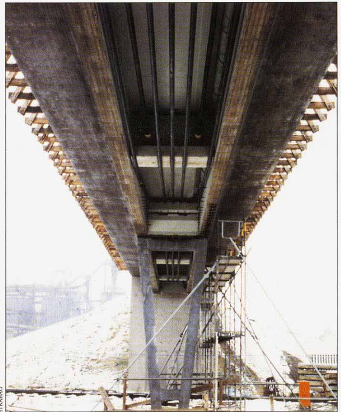
External Polystal prestressing tendons used in a Berlin footbridge.
