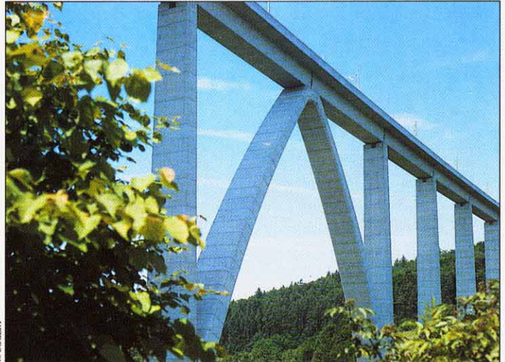
The 'A frame' portal provides the only fixed point in the 1 km long bridge.
