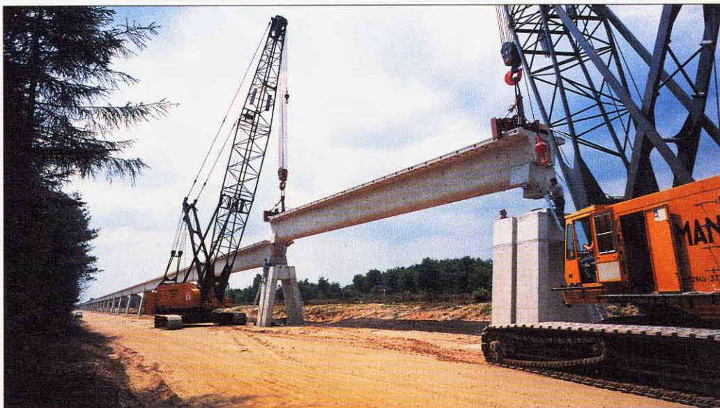
Erection of a prestressed concrete track beam.
