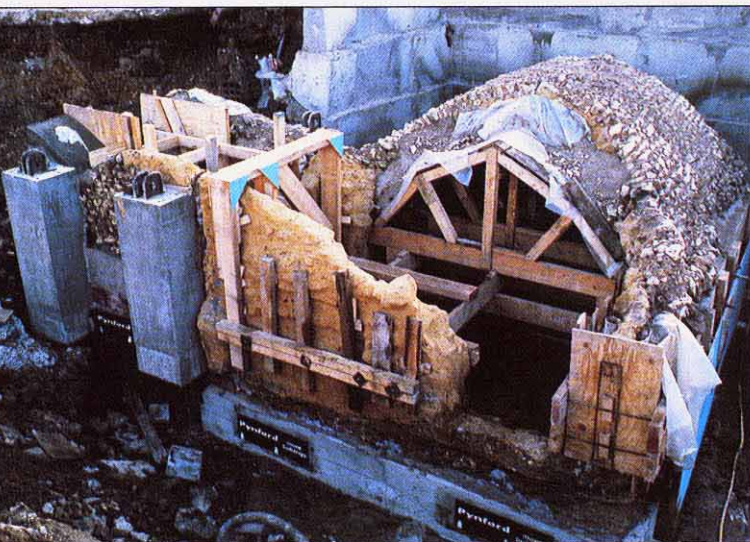
The staircase and undercroft, strengthened and underpinned.
