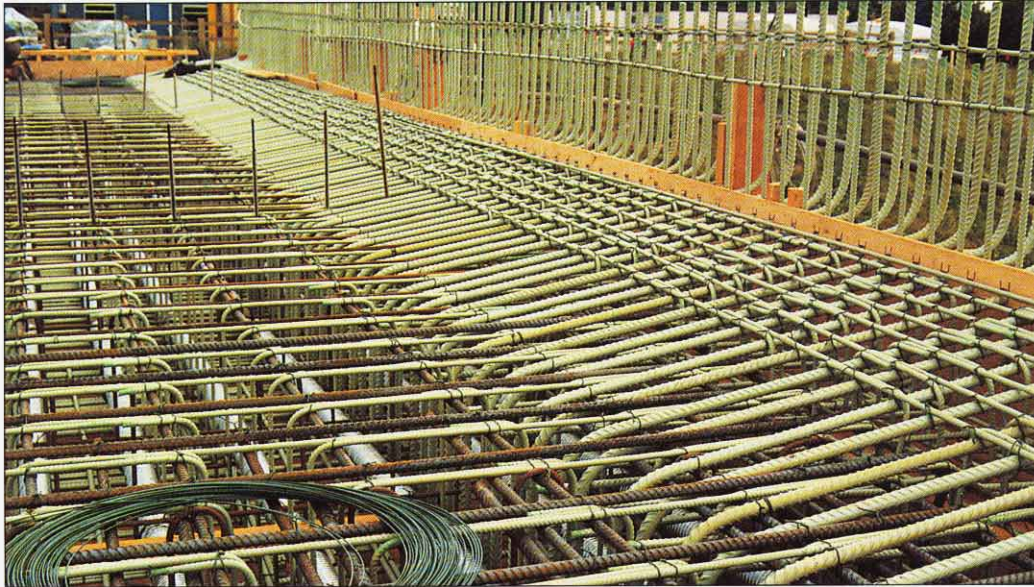
Epoxy coated reinforcement in a bridge recently built for British Rail near Reading. The soffit will be exposed to salt-laden spray.
