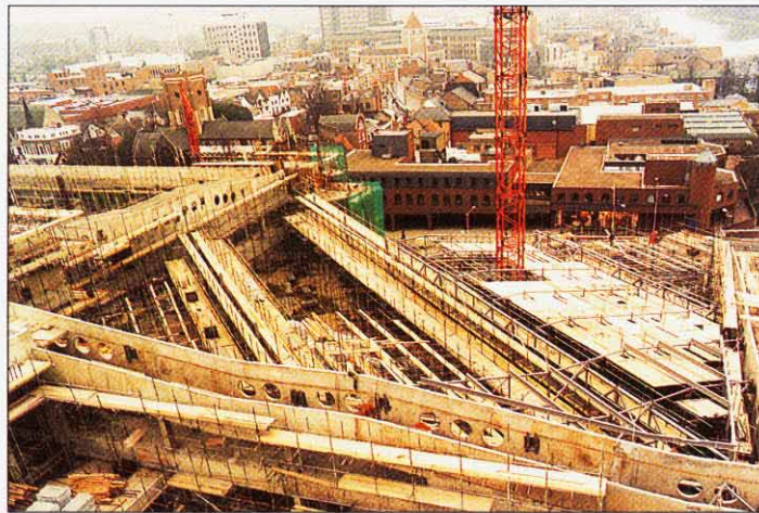
A 2 m square plenum runs round the perimeter of the roof.
