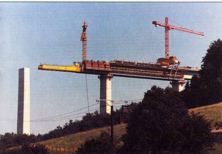
Superstructure beams were cast in a prestressed concrete self-launching girder.
