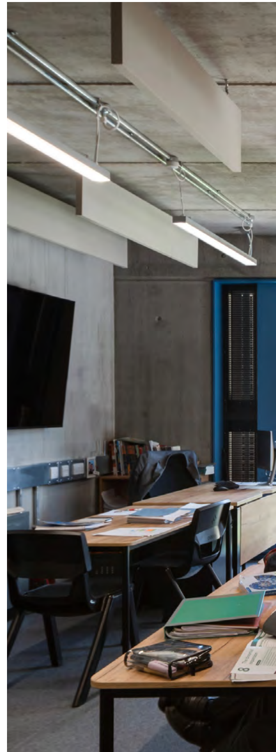
ABOVE At Levitt Bernstein's recently completed building for Eltham College in south-east London, the precast-concrete structure is exposed internally to exploit the thermal mass and provide a contemporary contrast to the school's historic quad. In classrooms, acoustic baffles are hung vertically to maximise the area of soffit exposed to cross-ventilation
