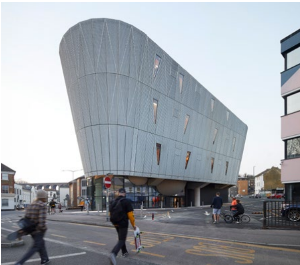
TOP The bowls rest on perimeter columns, leaving the cafe column-free ABOVE The building is unheated and simply covered in an aluminium mesh
