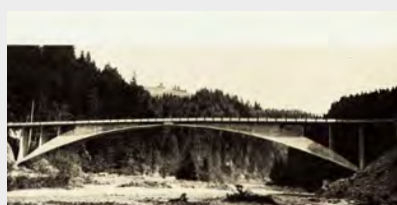
The slenderness of Birsingen-bridge, near Schwanenried, is made the more apparent by its light open girders.
