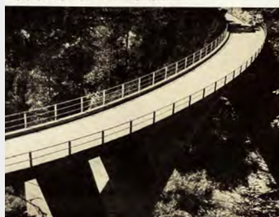
Schwanenried bridge built in 1904 is now faster than the Birsingen bridge, on the same road. Executed on a curve, with a span of 125 ft, this bridge is one of Maillart's most brilliant engineering achievements.
