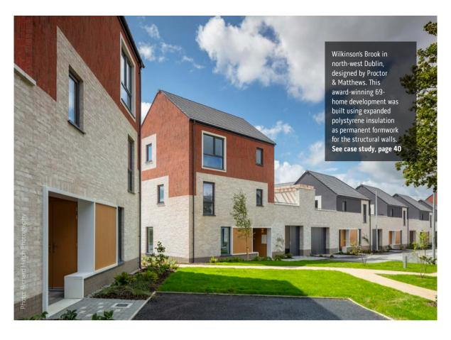
Insulating concrete formwork for low-rise housing
