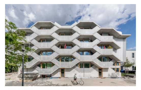
room is 6.6m across the centre. The once-vertical walls slope outwards at a 160° angle before doubling back on themselves. Bespoke slanting furniture climbs the walls, effectively extending the floor space. The larger apartments are split, mezzanine-like, over 1.5 levels with openings in the lower wall that step down to the adjoining cell. "You can combine the spaces as you like," says Haimerl.
