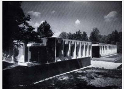
Below: The most striking feature of the office block, showing the way the precast concrete columns are joined together.
