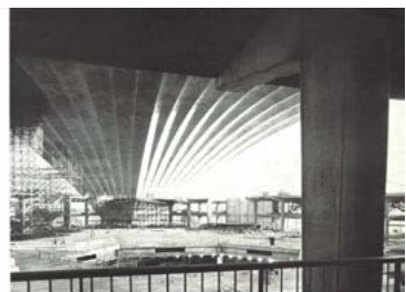
The roof was an immense precast concrete shell. The volume on the right supports the upper gallery, the centre is open to the hall below.
