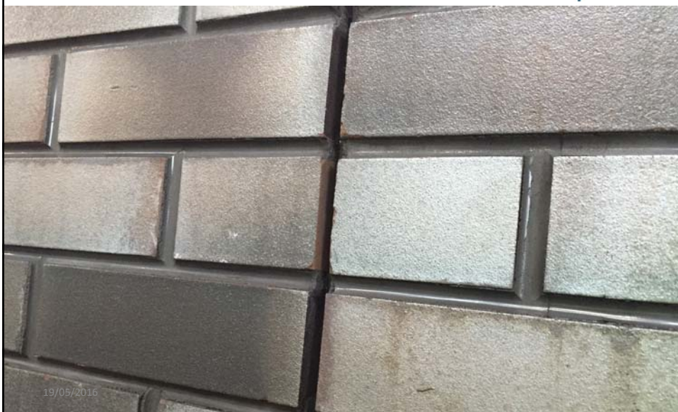
Detail: Joint size and location
