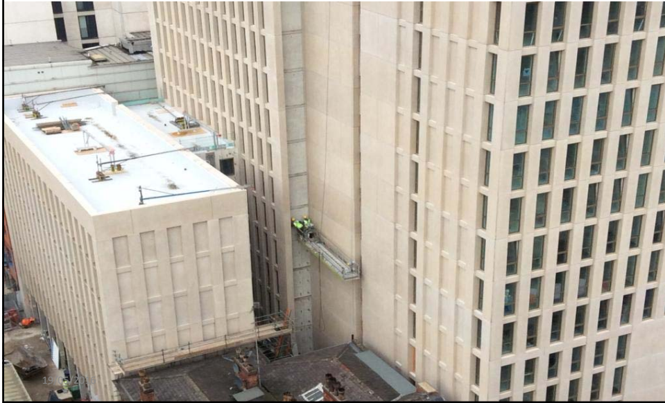
Acid etched precast concrete sandwich panels
