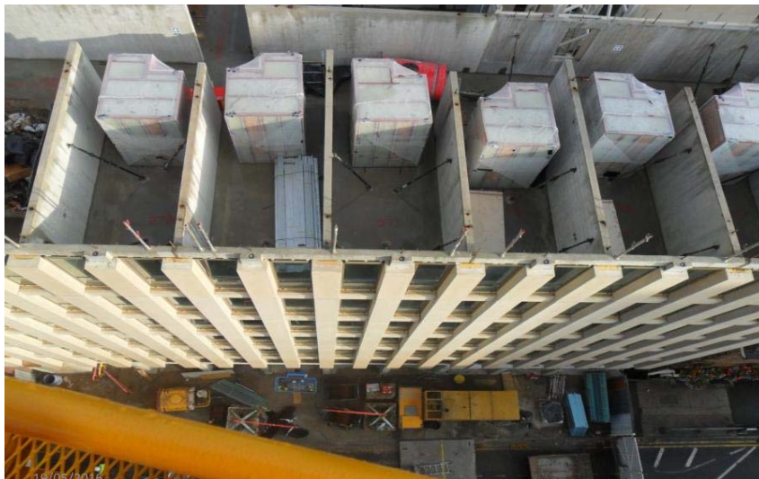
Cross wall, bathroom pods, insulated sandwich panel facade
