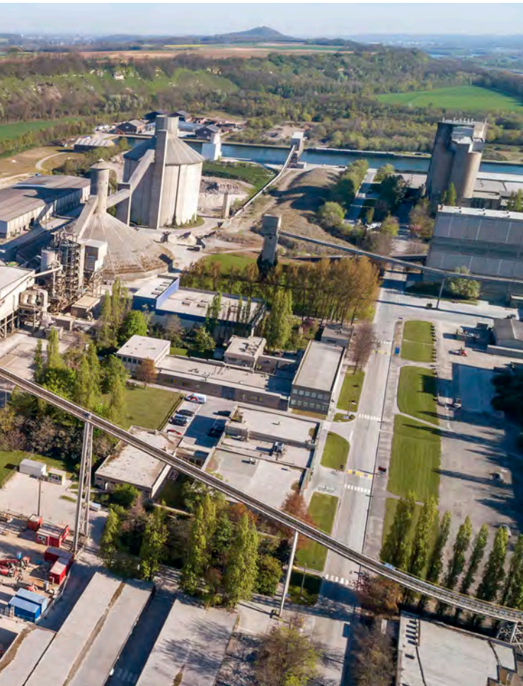
ABOVE The LEILAC project has been testing the application of “direct separation” technology to the cement and lime industries at the HeidelbergCement plant in Lixhe, Belgium
