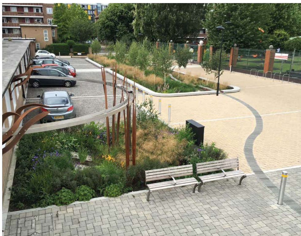
Opposite and right: Bridget Joyce Square in west London, where Robert Bray Associates has installed a community rainpark with concrete block permeable paving laid over the existing concrete road slab
