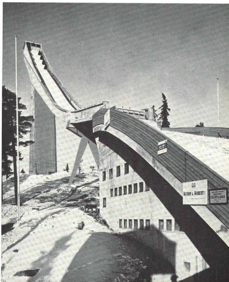
A closer view of the structure, showing the restaurant and museum building fitted in beneath it.
