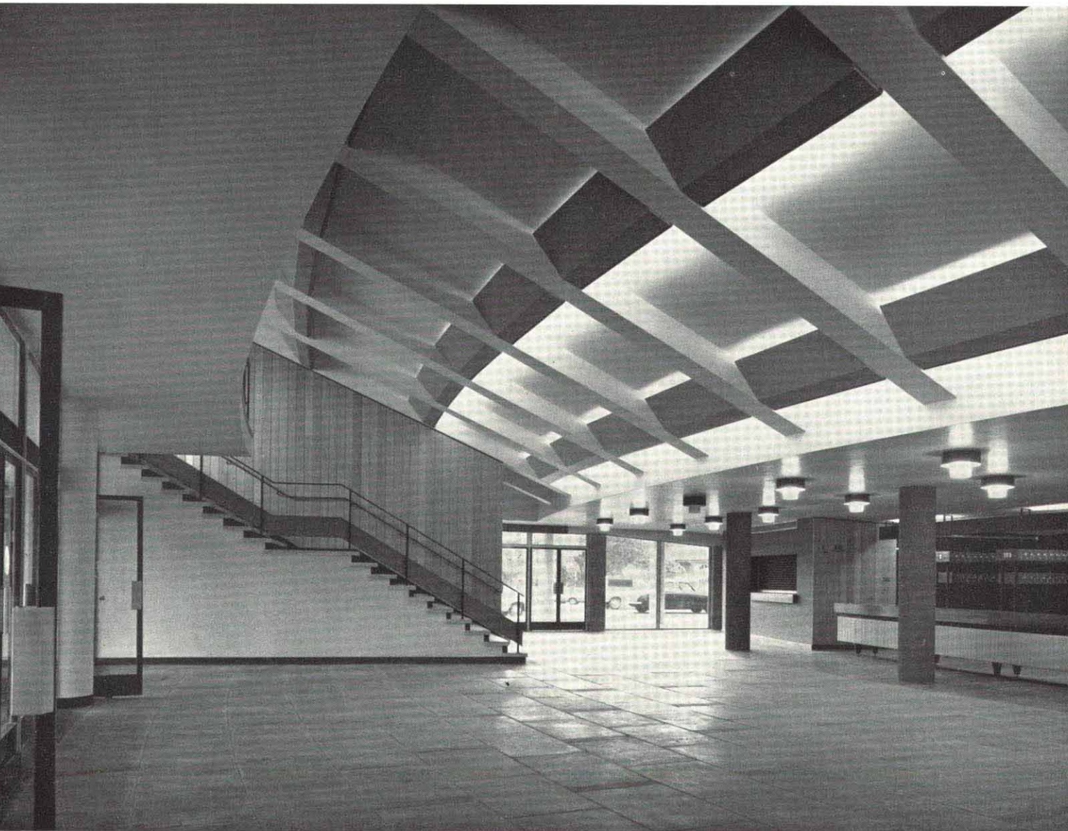
Above: The entrance foyer, paved with standard precast concrete flags.
