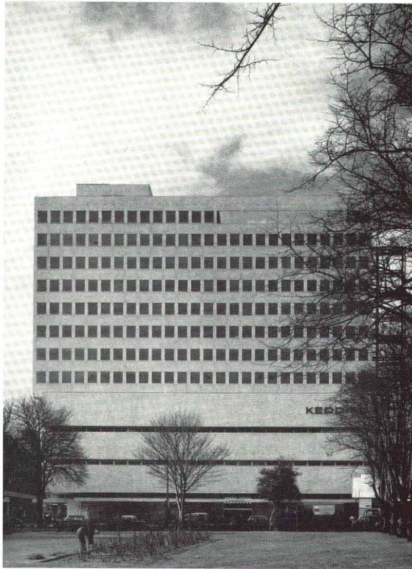
The lower sales floors of Keddies store are lit by narrow strips of windows. Offices are housed in the eight floors above.
