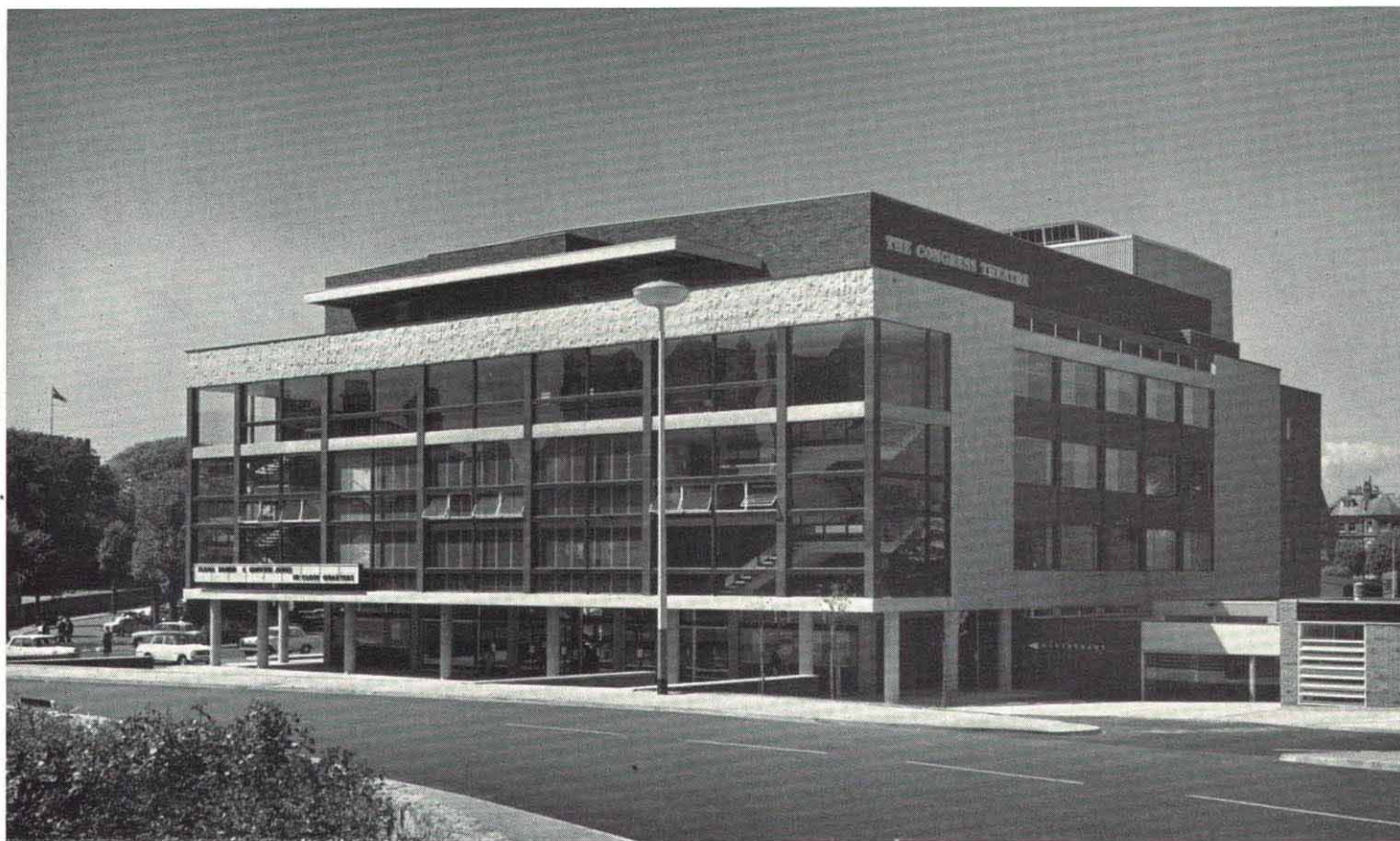
White riven 'Maclit' blocks form a continuous band along the front and sides of the theatre.
