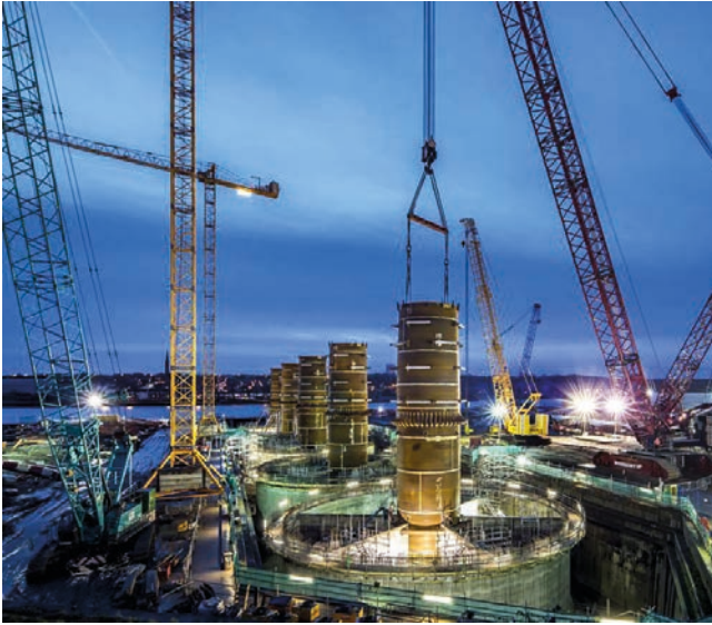
Above Turbine substructures under construction. Each can weigh up to 20,000 tonnes
