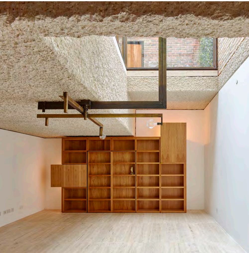
LEFT 21 Caroline Place in London by Amin Taha Architects. The soffit of this in-situ concrete basement were bush-hammered to create an unusual, rough texture. The mix combined a
