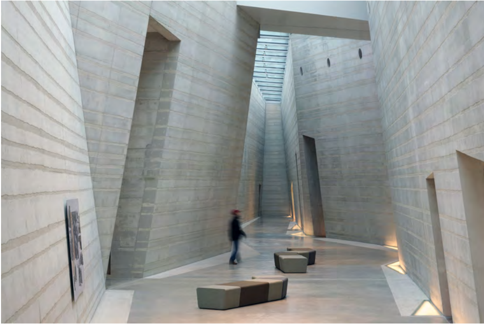
IN SECTION The visitor centre rises and twists with the hillside. Snøhetta describes the central circulation area as a “cut in the landscape”
