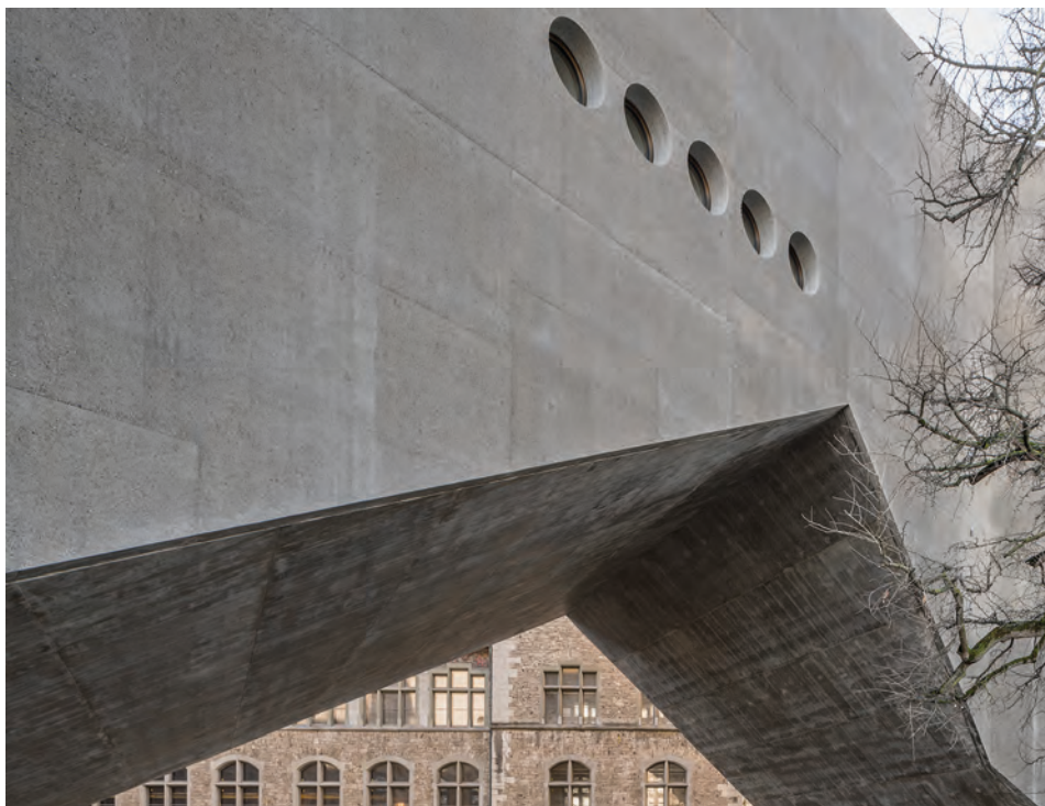
ABOVE Christ & Gantenbein's extension to the Swiss National Museum in Zurich. The external concrete contains a proportion of fly ash as a cement replacement, which darkened the tone and reduced the water content
