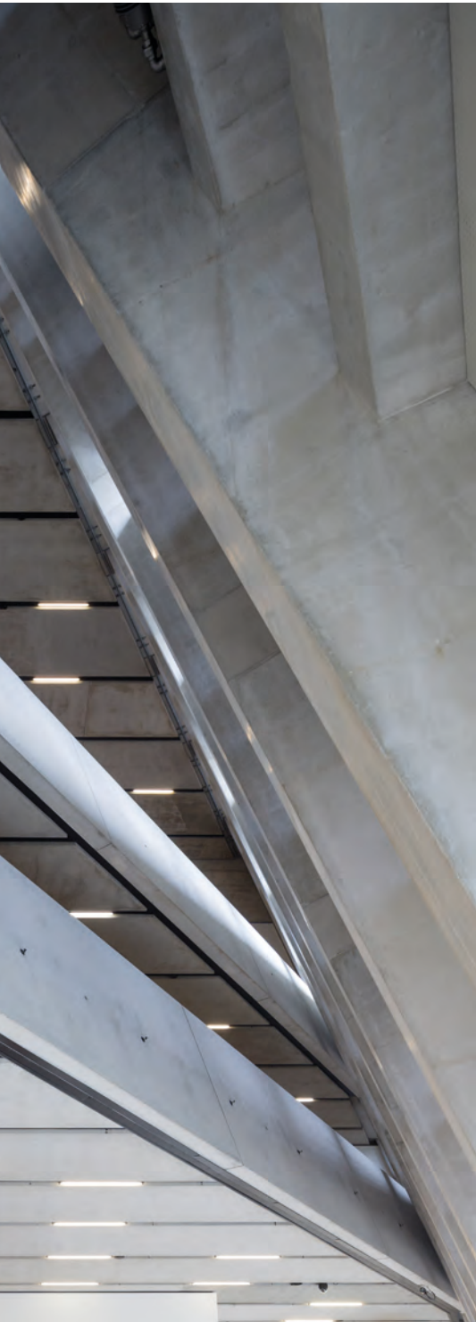
ABOVE The Switch House at Tate Modern, London, where a pale concrete containing 50% GGBS was specified
