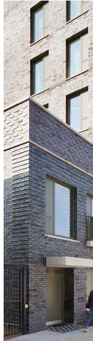
ABOVE The first phase of Agar Grove, a 38-unit apartment block designed by Hawkins\Brown, was completed in 2018
