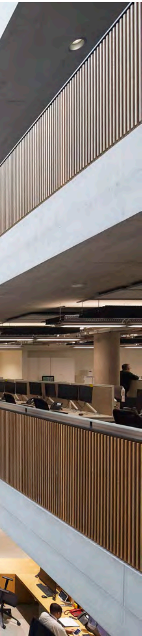
ABOVE The central atrium, where the in-situ concrete 10m-grid structure is clearly visible
