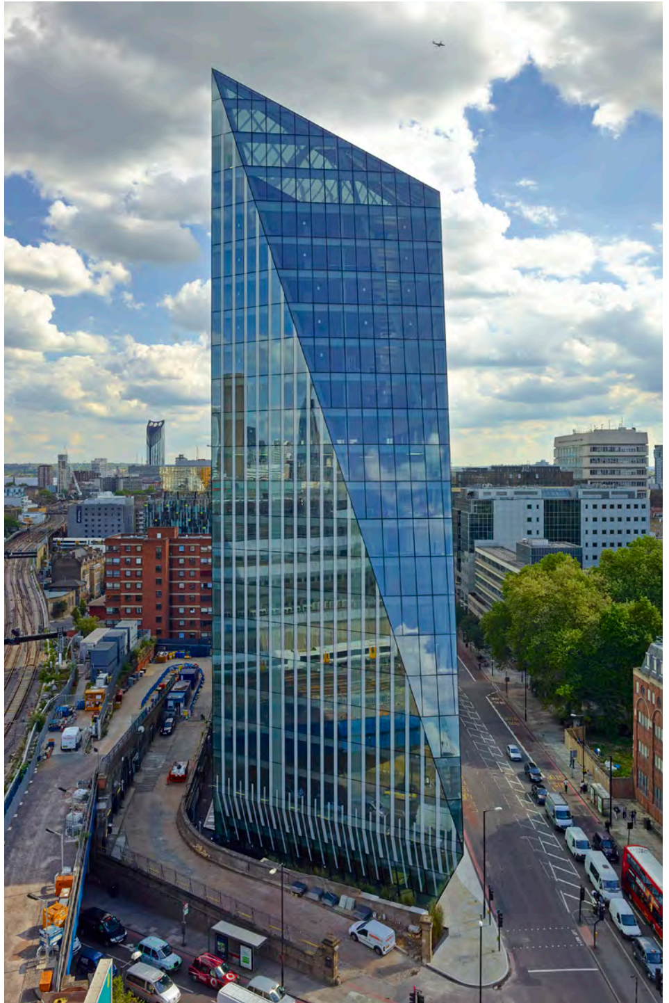
RIGHT At 240 Blackfriars Road in London, the use of PT slabs enabled architect AHMM to add two storeys without increasing the building height
