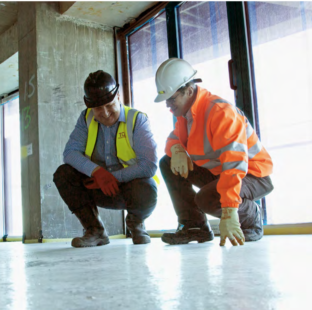
ABOVE Surface regularity of screeds is classified under BS 8204-1, and specified by quoting classes SR1, SR2 or SR3
