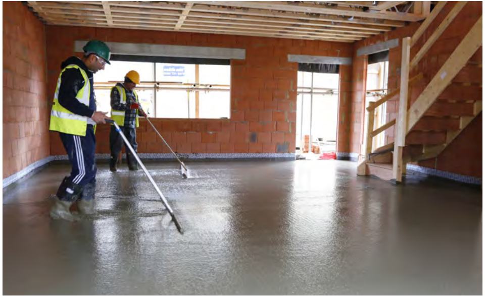
ABOVE Self-smoothing screed being laid at the low-energy Wienerberger e4brickhouse at the BRE Innovation Park in Watford
