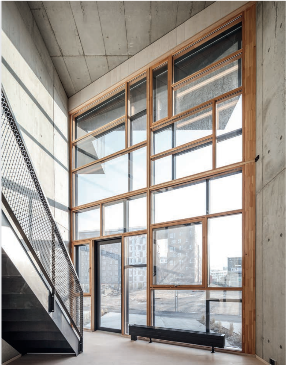
ABOVE In all, 837m 3 of upcycled concrete was cast in the construction of Upcycle Studios
