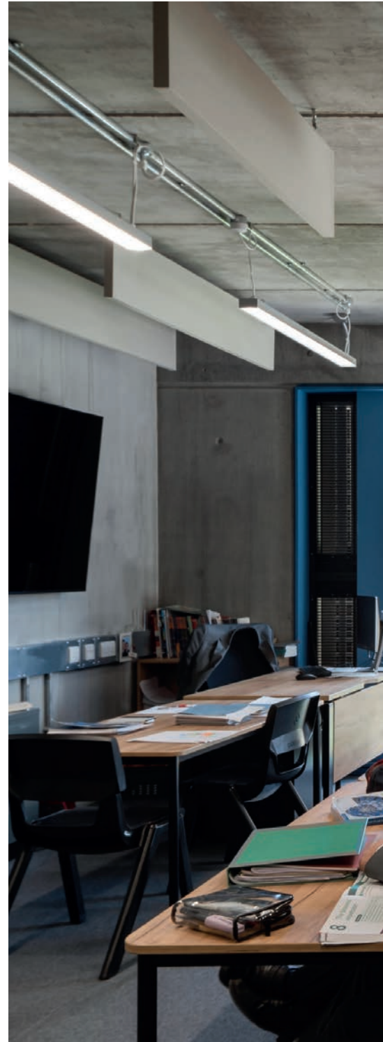
ABOVE At Levitt Bernstein's recently completed building for Eltham College in south-east London, the precast-concrete structure is exposed internally to exploit the thermal mass and provide a contemporary contrast to the school's historic quad. In classrooms, acoustic baffles are hung vertically to maximise the area of soffit exposed to cross-ventilation
