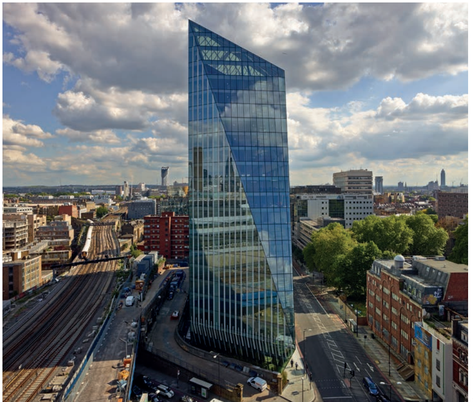
ABOVE At 240 Blackfriars Road in London, the use of PT slabs enabled the addition of two storeys without increasing the building height
