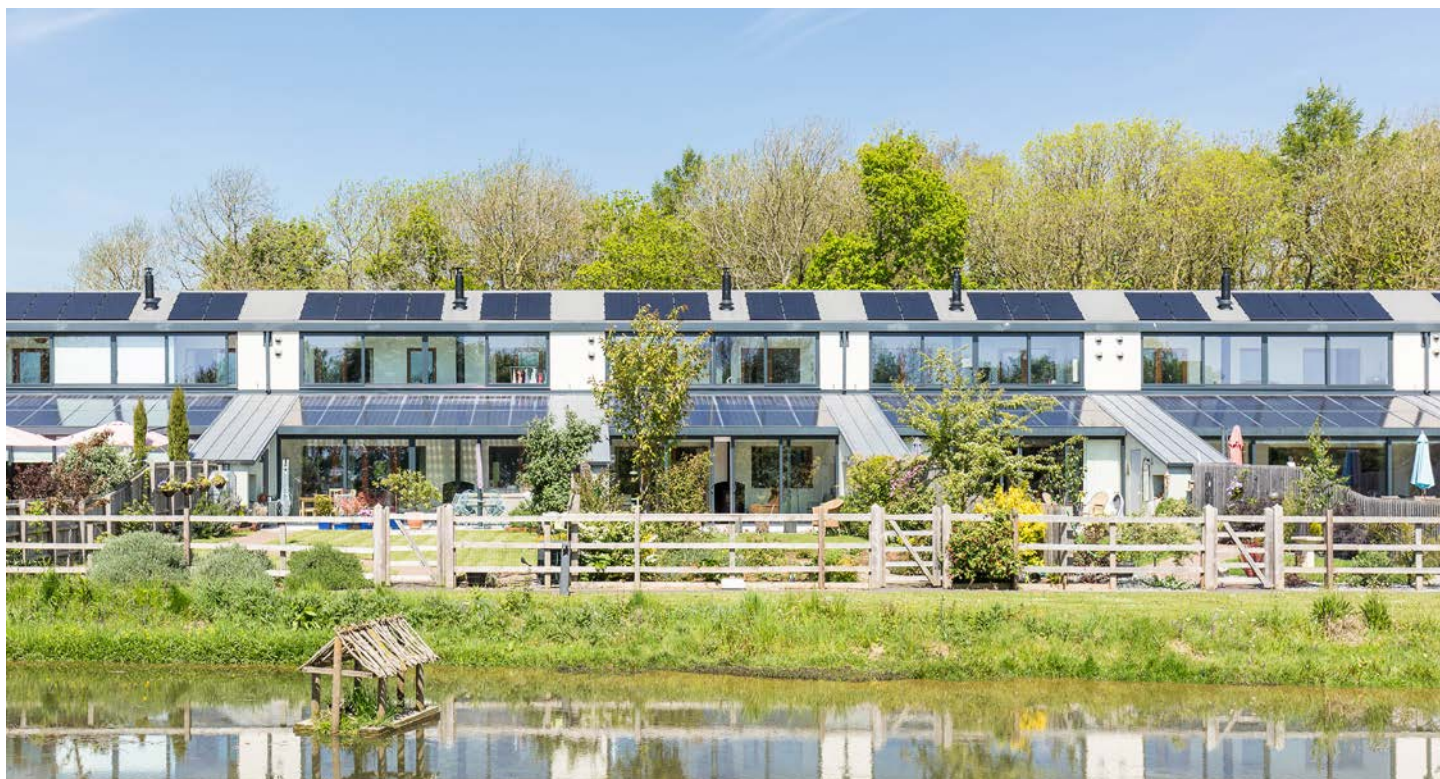
ABOVE Gusto Homes' Woodlands Edge development near Lincoln. The majority of glazing is on the south side, maximising solar gain and minimising heat losses from north-facing elevations
