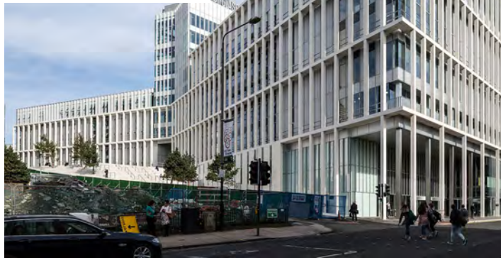
Photos: Keith Hunter; Jeff J Mitchell/Getty Images; KAZA Concrete; Paul Osborne/Compound Eye
