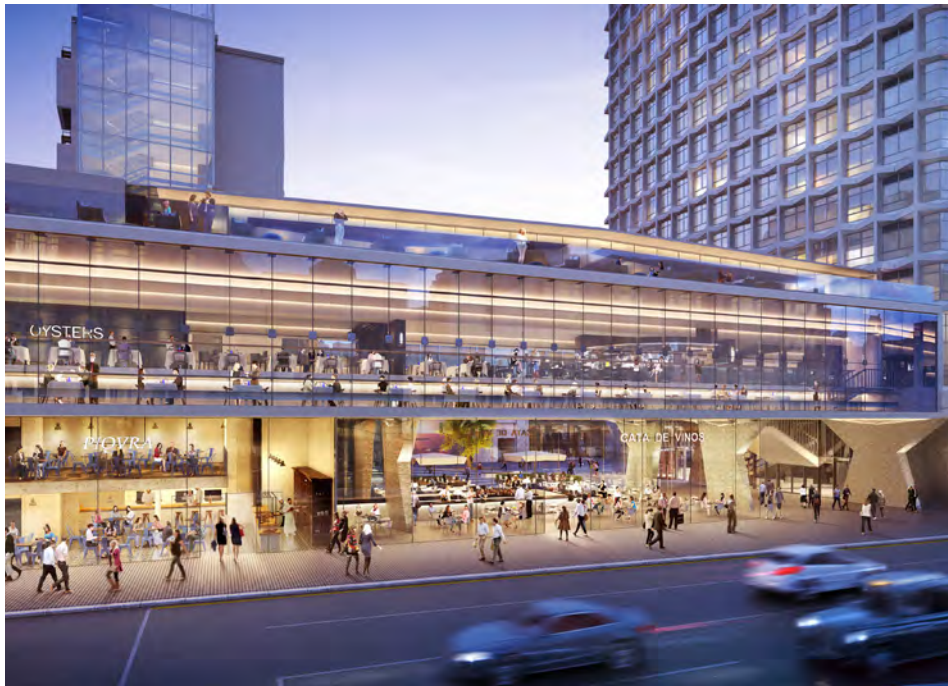
ABOVE A lightweight glazed infill is being inserted below the bridge link
