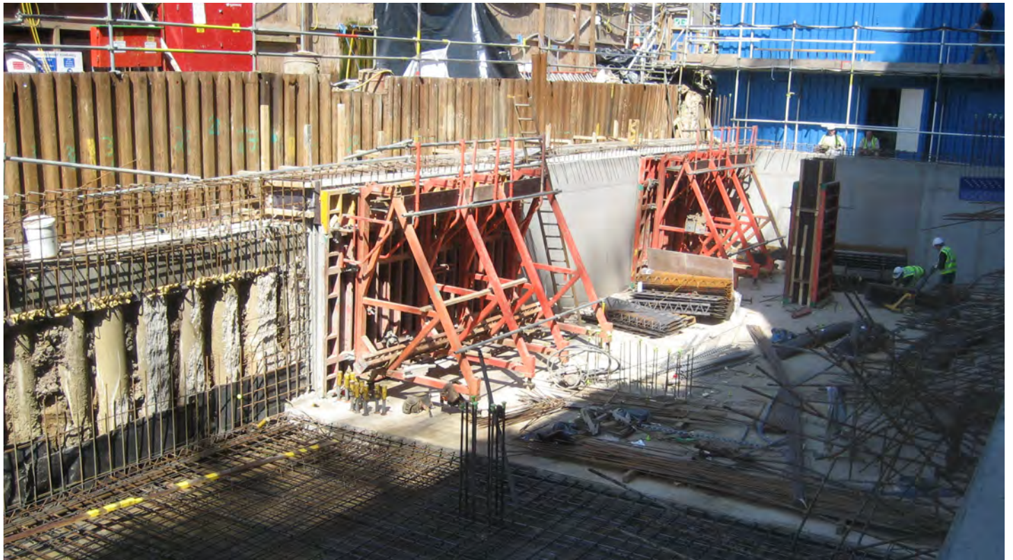
ABOVE Facing wall to a contiguous piled wall
