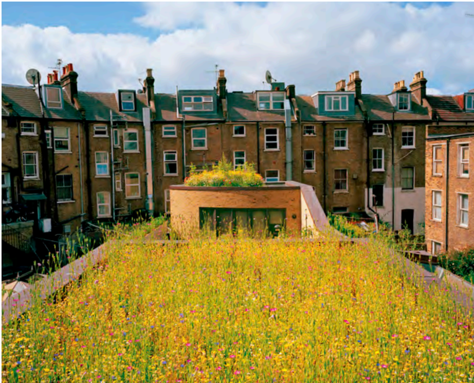
ABOVE The Muse, a family home in Islington, north London has a green roof with varying soil depths for native habitats, including two wildflower meadows, a hazel coppice and a hawthorn thicket
