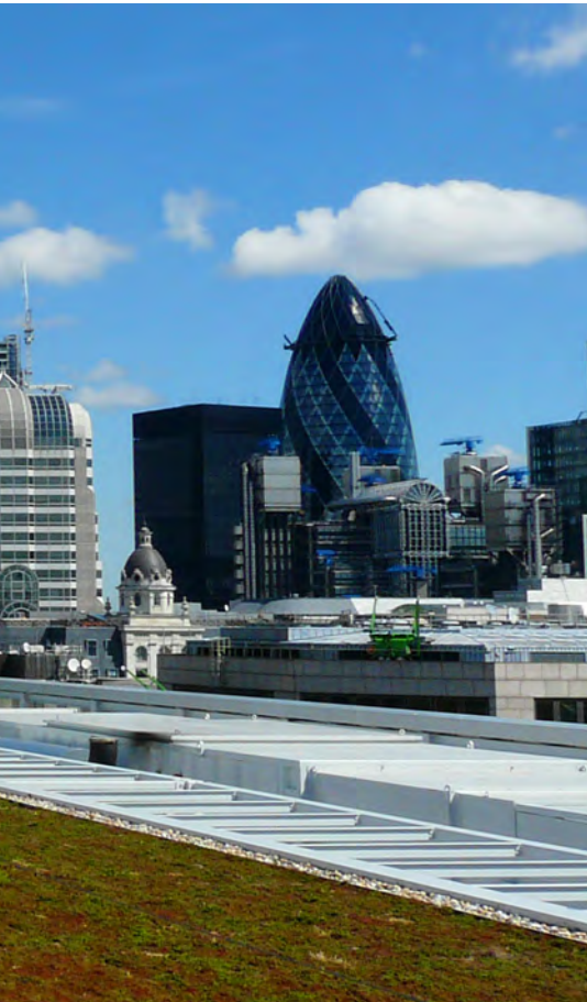
ABOVE Riverbank House in the City of London has an extensive green roof planted with sedum
