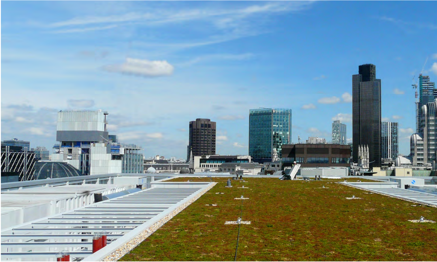
Photo: Courtesy of IKO PLC
