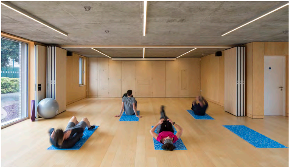
ABOVE The in-situ slab at PAD Studio's Canoe Lake tennis pavilion in Portsmouth was poured in one go using phenolic-faced ply formwork
