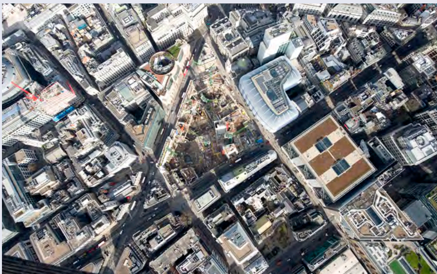
ABOVE At Foster + Partners' Bloomberg London, winner of 2018's Stirling Prize and one of the world's highest-scoring BREEAM rated office buildings, the concrete in the piles contained 100% recycled granite aggregate. This is classified as a secondary aggregate and is a by-product of the china clay industry in Devon and Cornwall
