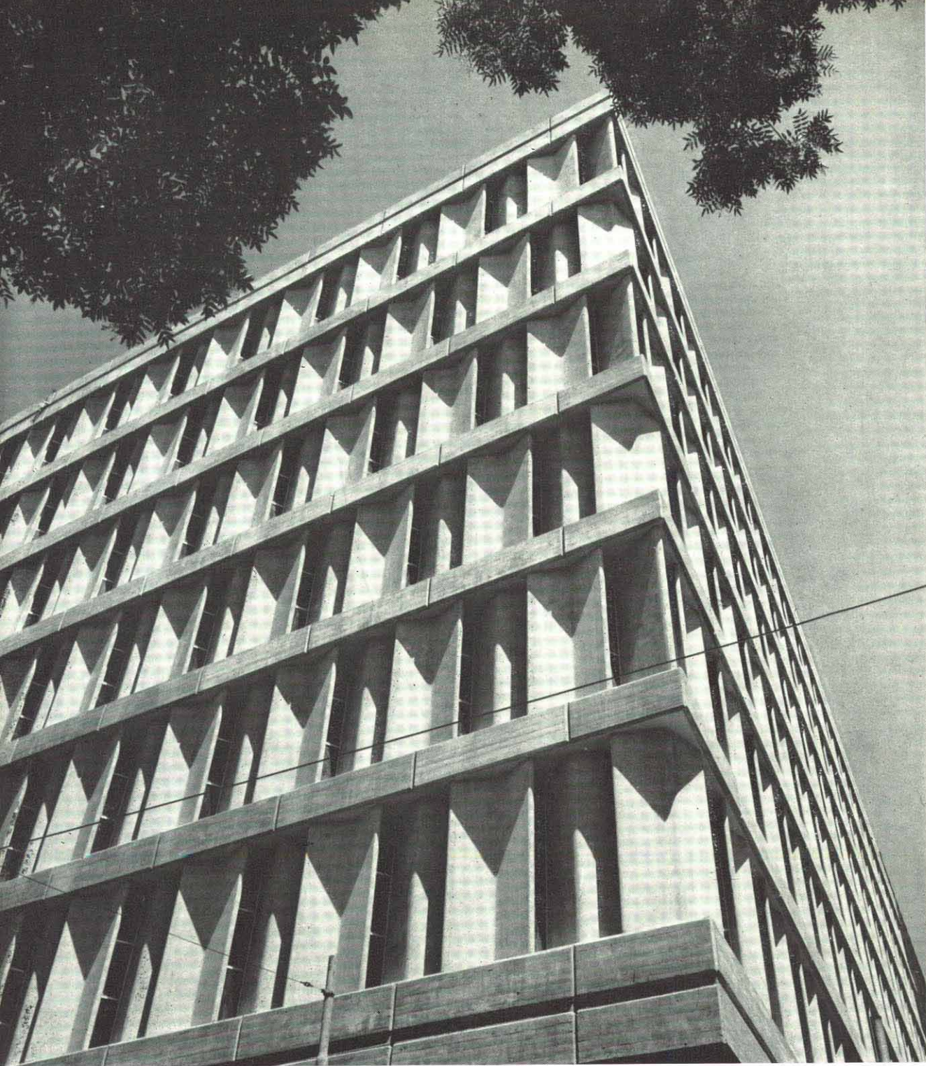
Prefabricated brise-soleil facade, IBM Building, Madrid (see also front cover).
