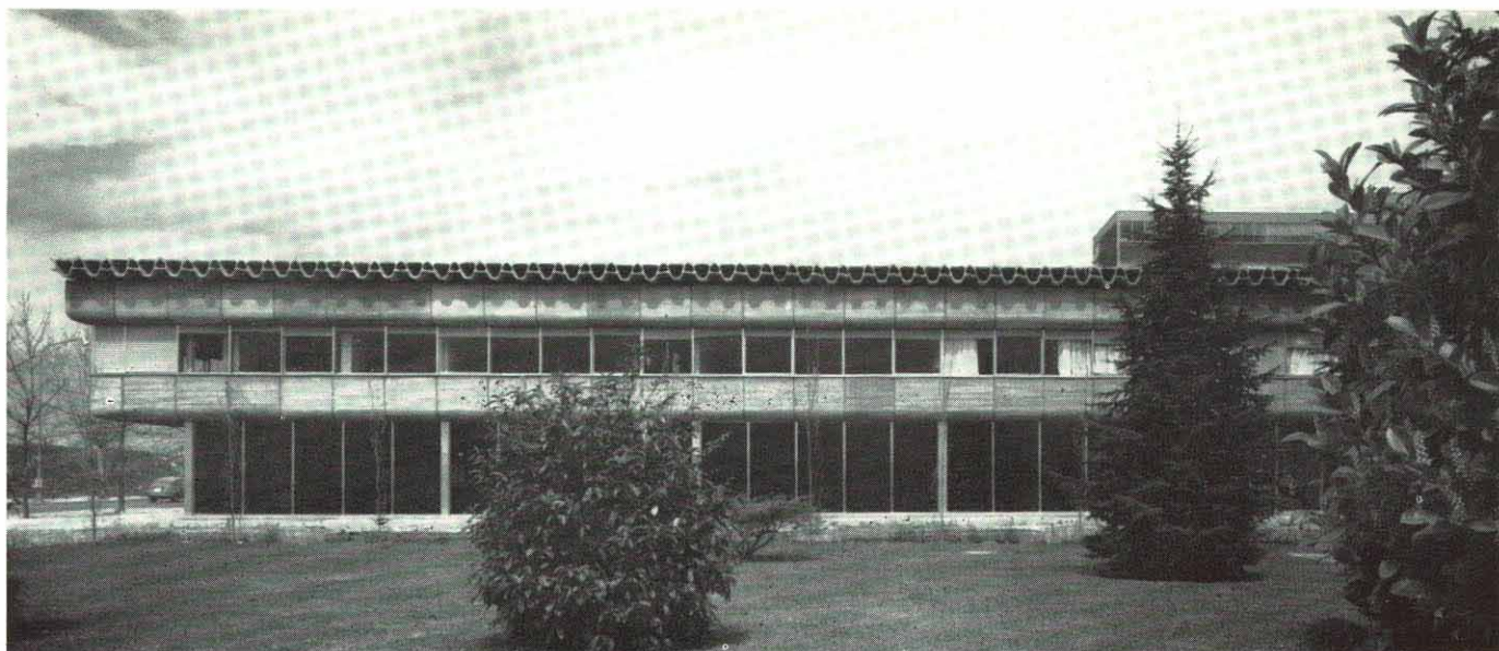
Electricity Building, Madrid.
