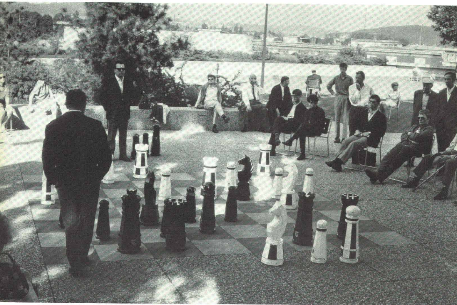
A chess game on the roof of Berne station. Black and white exposed aggregate slabs are used with 'Washbeton' slabs round the perimeter.
