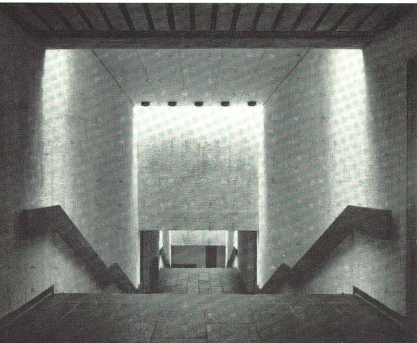
Above : Stairway in the Hotel Stavrbj Skov, connecting bedrooms with vestibule. Floor and stair of black slate, wall finishes of heavily rough-cast rendering unpainted.
