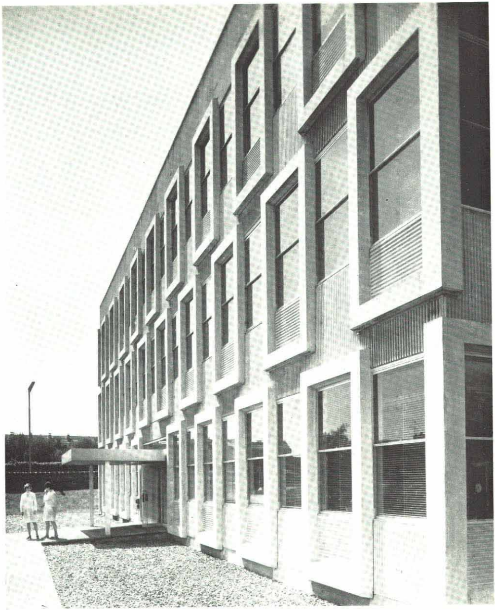
Oblique view of the front elevation showing in detail the Laing wall frames and the ribbed concrete.
