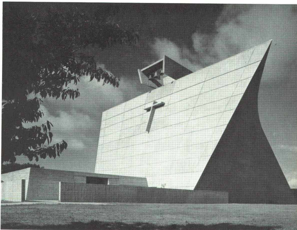
View of the church from the north-east, showing one of the oversailing hyperbolic paraboloid side walls of the nave (in shadow). The rear nave wall, with the cross on it, is an inclined flat plane.
