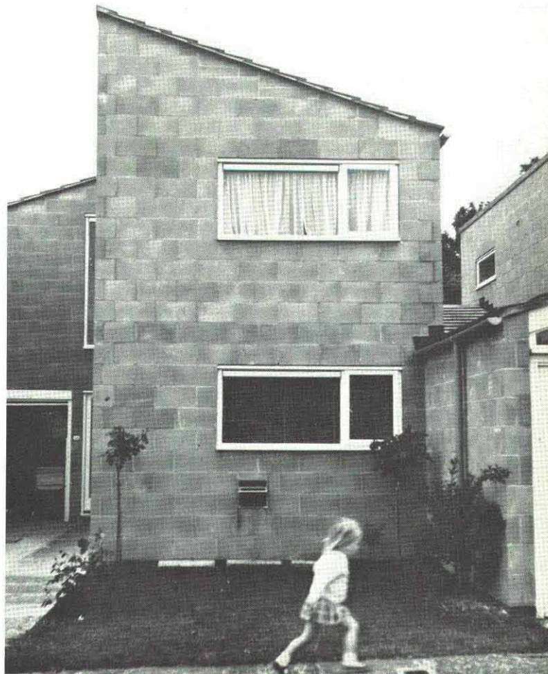
Elevation of one of the Shrublands houses. Note the liveliness given to wall surfaces by the slight colour variation in the blocks.
