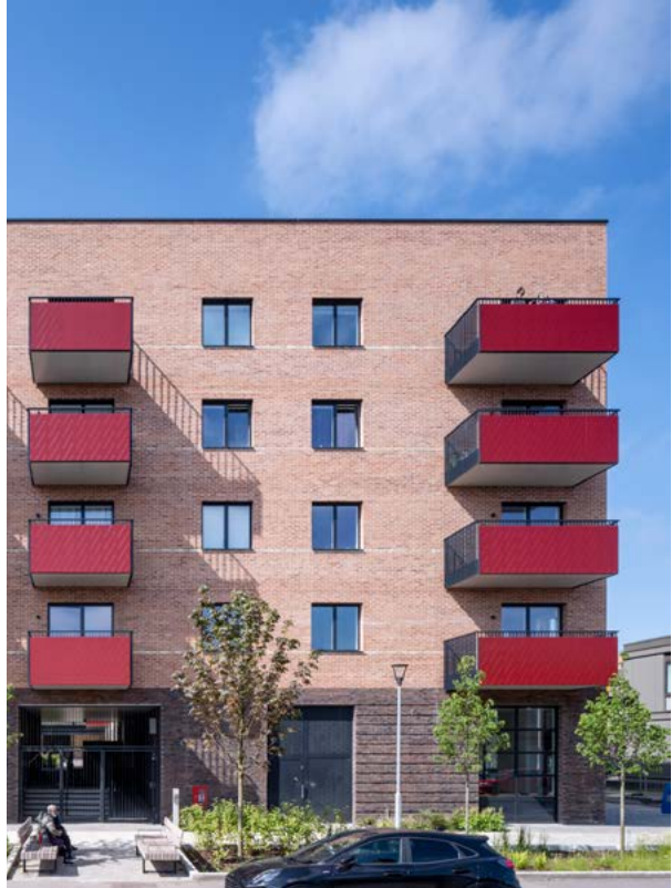
ABOVE The facade features three different shades of hand-laid brick and striking red metal balconies
