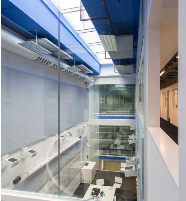
ABOVE LEFT The painted concrete soffits are a blue of 480nm spectral wavelength, chosen for its effect on mental alertness
