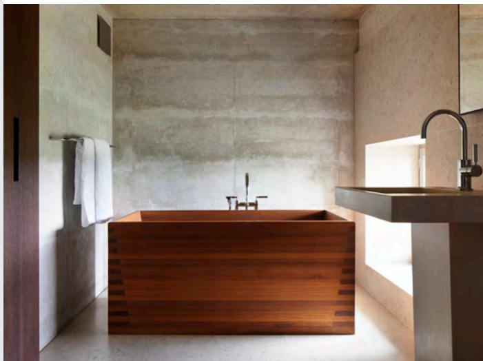
ABOVE The rammed-concrete walls at Secular Retreat are 750mm thick: two 300mm layers of concrete encase 150mm of insulation
