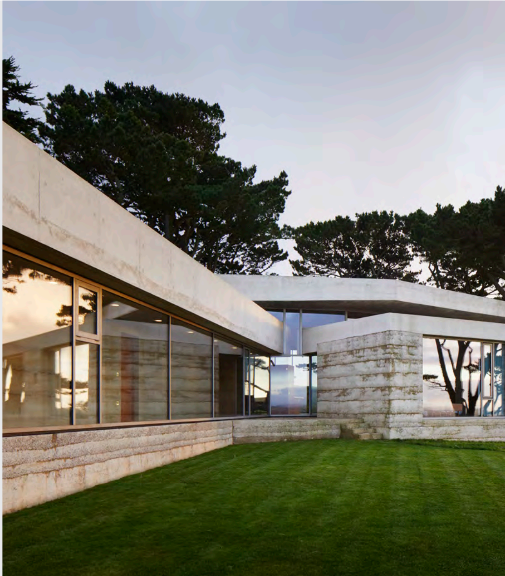
ABOVE The rammed-concrete walls at Secular Retreat are 750mm thick: two 300mm layers of concrete encase 150mm of insulation
