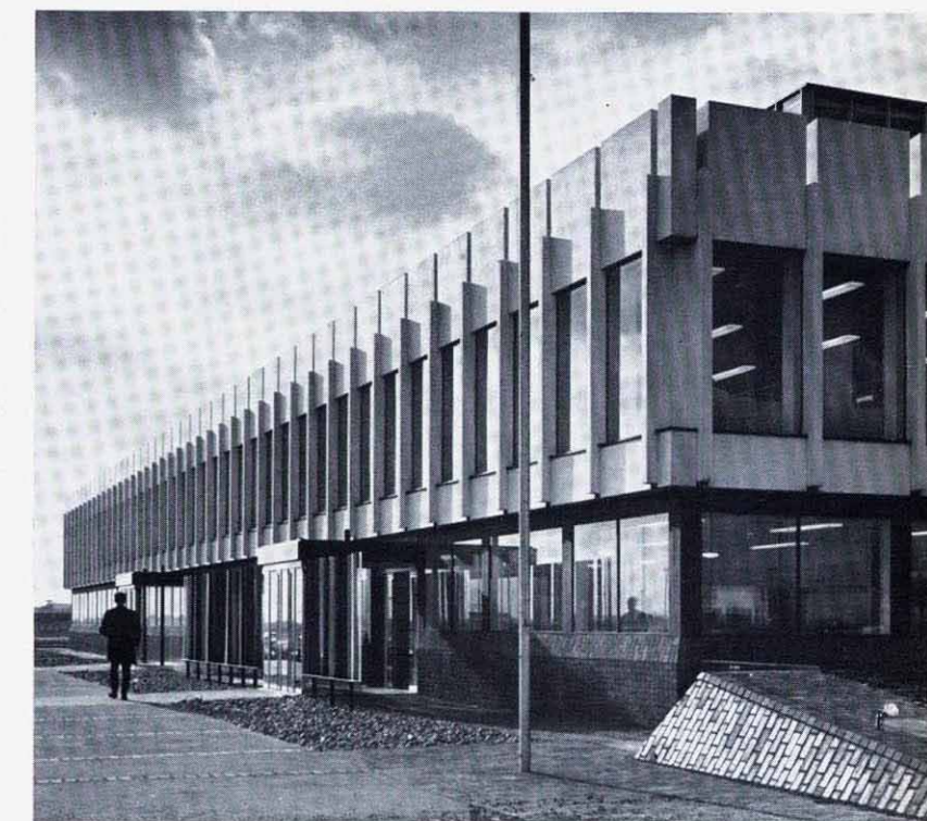
Oblique view of the Custom House from the broad paved terrace.
