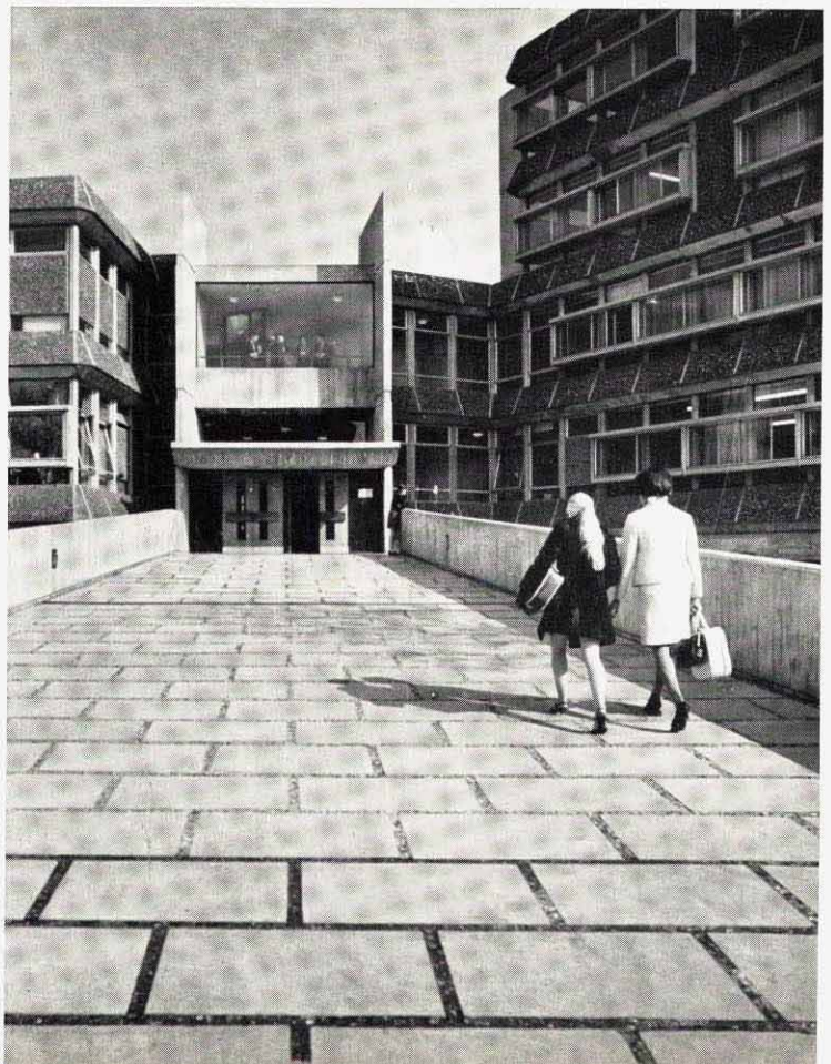
The main entrance approach. Note the wide flint-filled joints between paving slabs.
