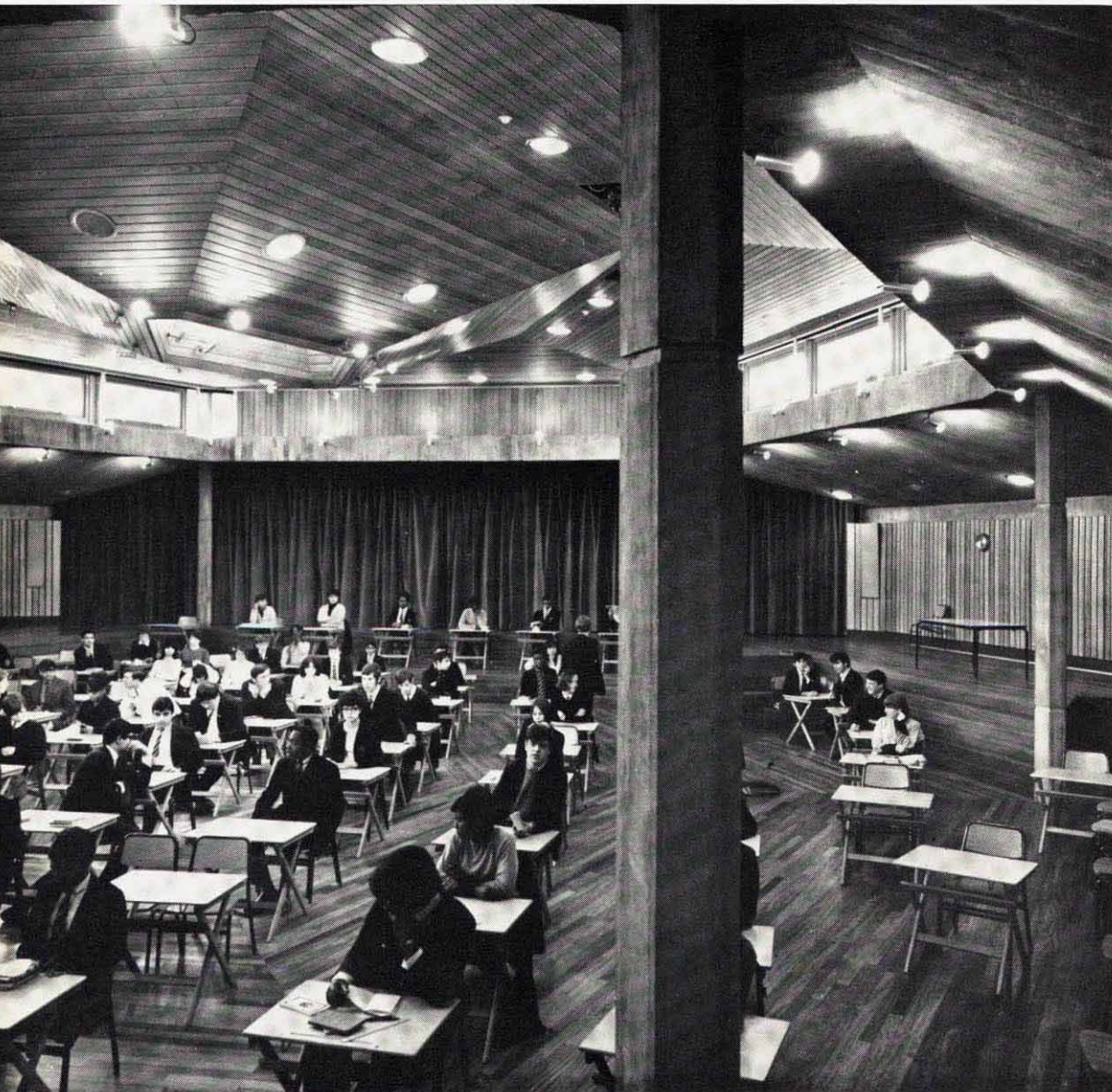
Exterior and interior views of the assembly hall, Acland Burghley School.
