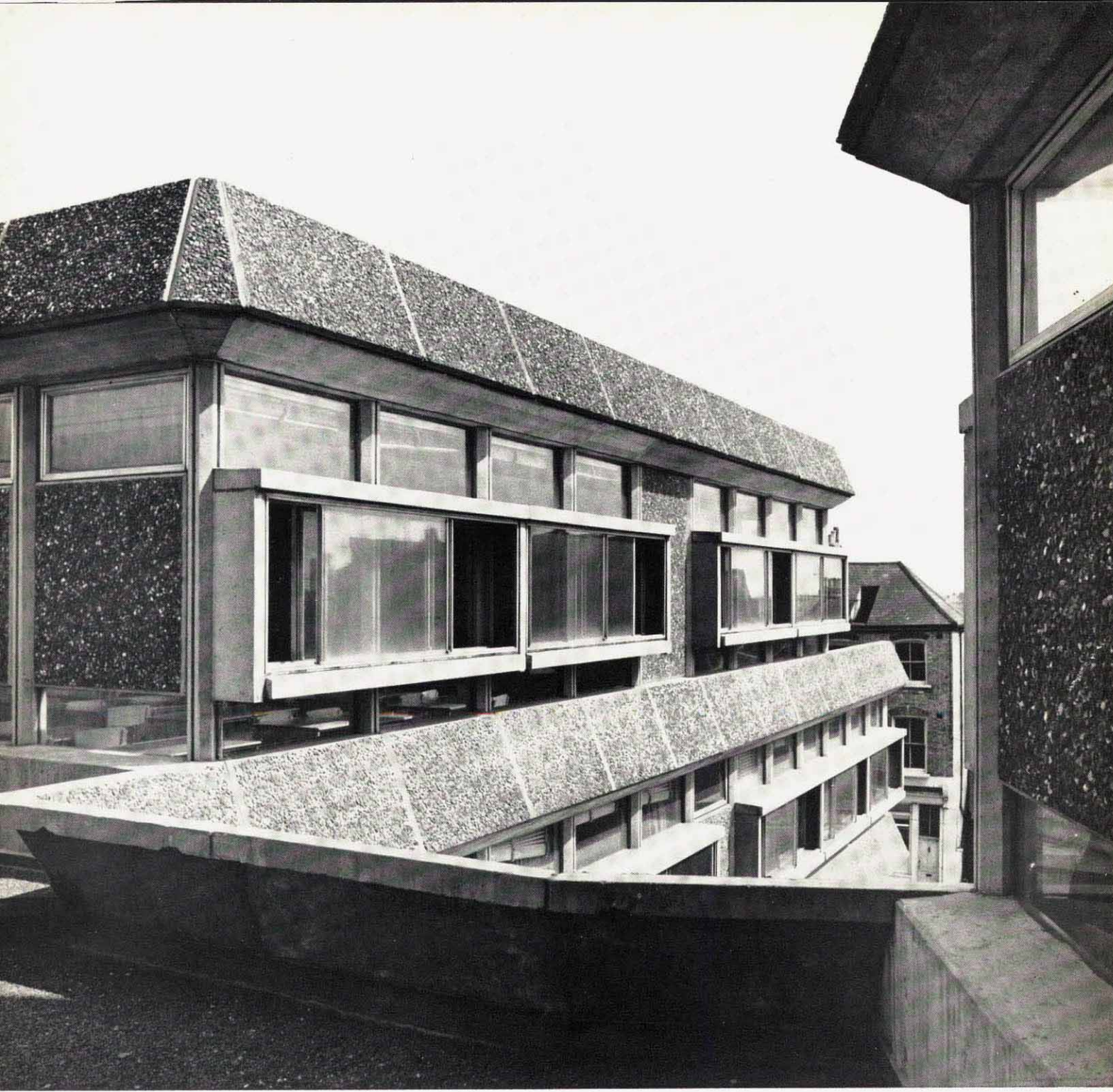
Detail of one of the classroom wings showing the modelling achieved by splayed cladding panels and projecting window.
