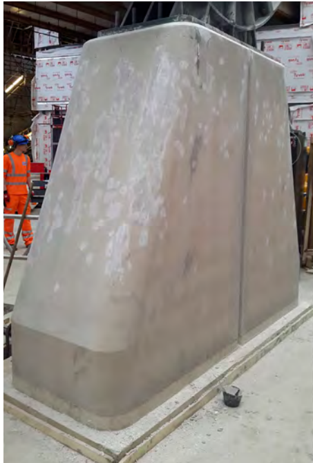
ABOVE The high-quality finish of the self-compacting concrete at London Bridge station's new concourse required some post-finishing
