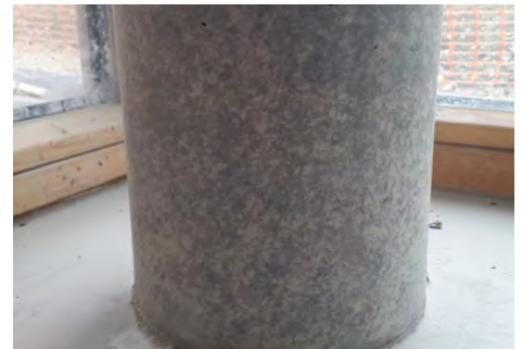
ABOVE An example of construction joint repair
