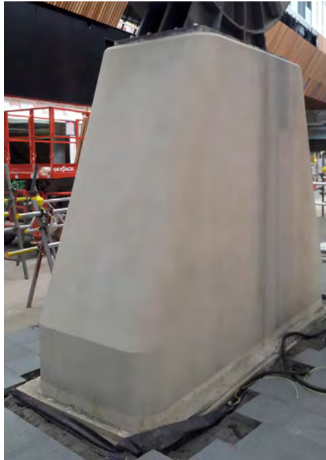
ABOVE The high-quality finish of the self-compacting concrete at London Bridge station's new concourse required some post-finishing
