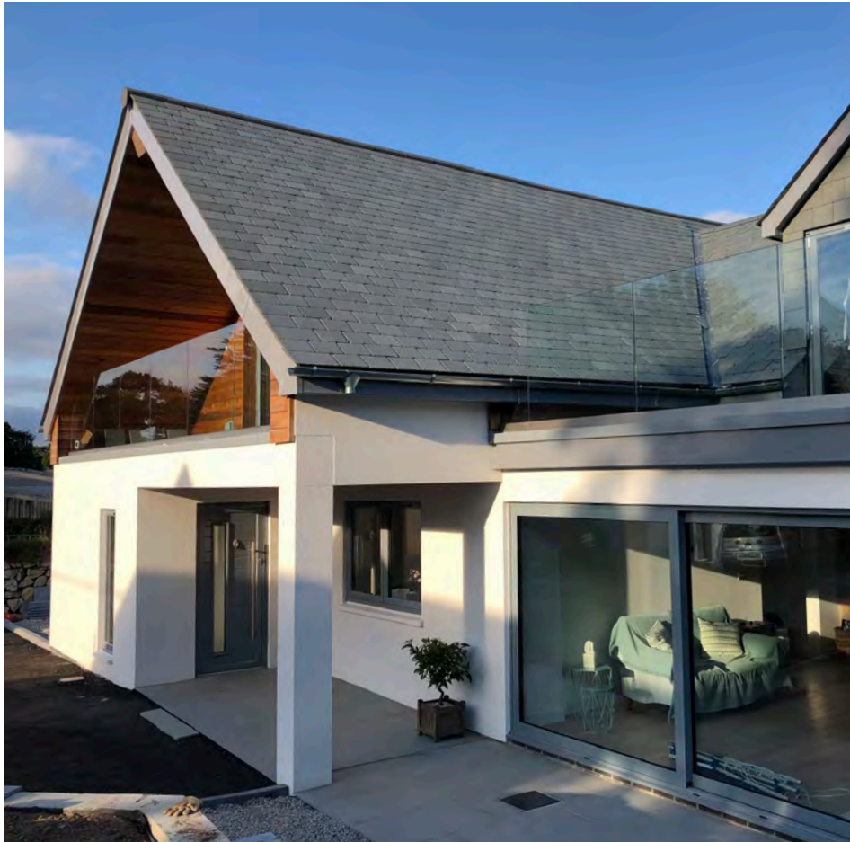
Photos: CCP, HexxHome, Tarmac, RoofSpace Solutions
