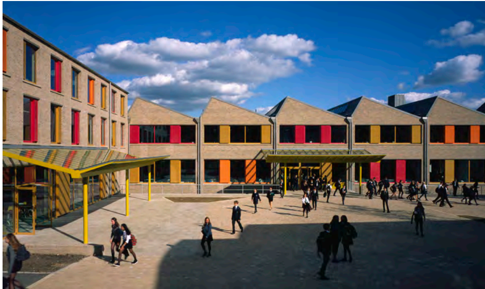
ABOVE Severn Oaks School Science & Technology Centre has a precast concrete roof in a sawtooth design with 7m spans
